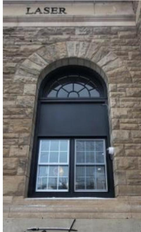
Figure 56: Detail of the front (northeast) elevation of the existing building at 78 Main Street South, showing the arched window opening with radial stone voussoirs (Town of Halton Hills 2025)
