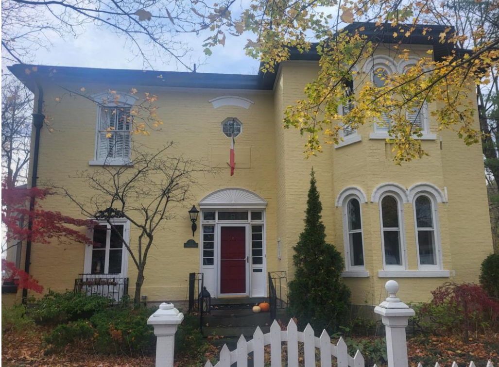
Figure 26: Front (northeast) elevation of the existing dwelling (Town of Halton Hills 2024)
