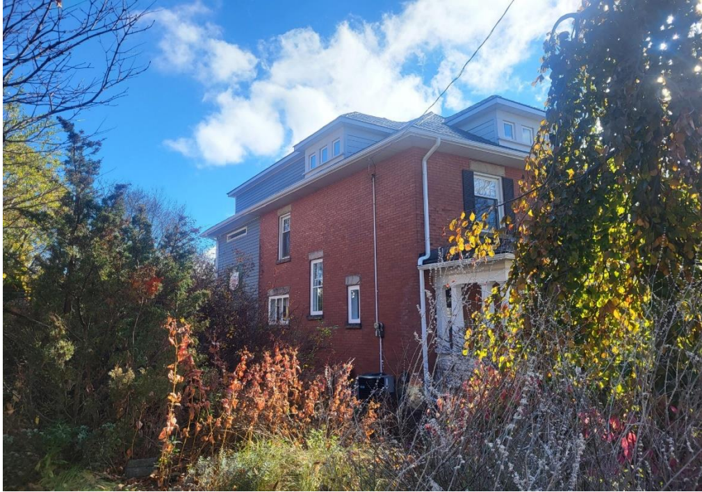
Figure 22: Side (northeast) elevation (Town of Halton Hills 2024)
