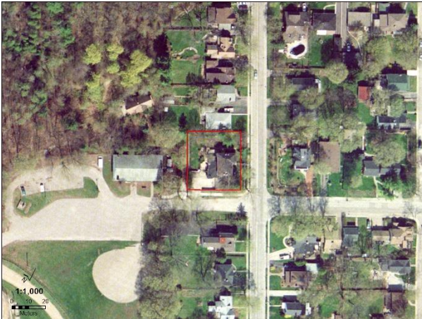
Figure 23: Subject property identified in 2002 aerial photography (Town of Halton Hills 2024)
