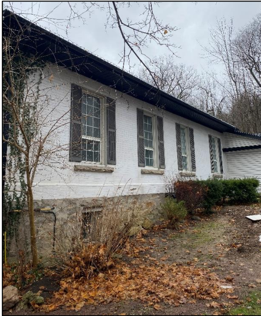
Figure 28: Side (northwest) elevation of the subject dwelling (Town of Halton Hills 2024)
