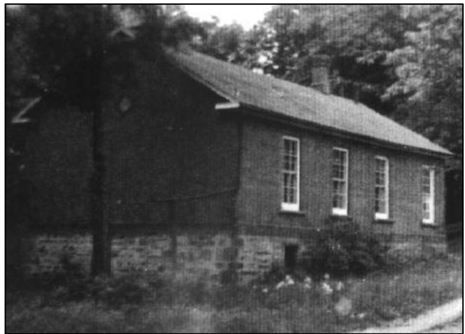
Figure 12: Front (northwest) elevation of Dufferin School, c. 1944 (EHS 11532)
