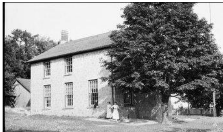
Figure 8: Exterior of Gibraltar Schoolhouse, c.1909 (EHS 19964)
