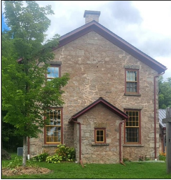
Figure 30: Front (southwest) elevation of the subject dwelling (Town of Halton Hills 2024)
