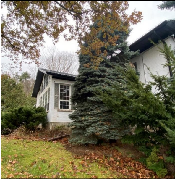
Figure 32: Side (southeast) elevation of the subject dwelling (Town of Halton Hills 2024)
