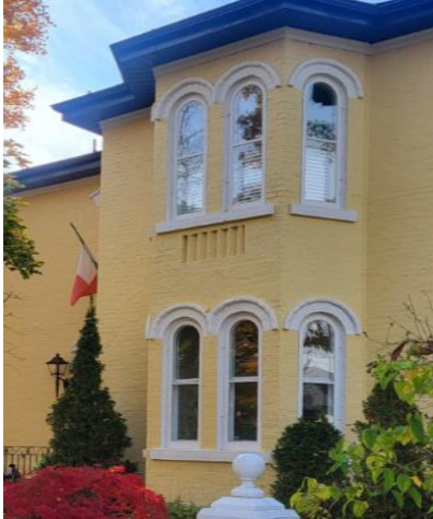
Figure 27: The projecting bay on the Front (northeast) elevation of 53 Charles Street (Town of Halton Hills 2024)
