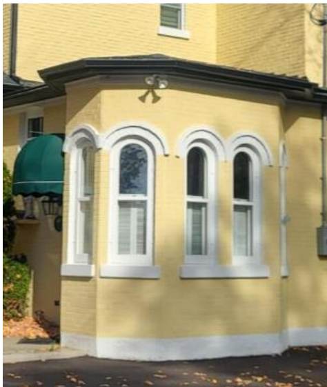
Figure 33: Projecting Bay on the southeast elevation of 53 Charles Street (Town of Halton Hills 2024)
