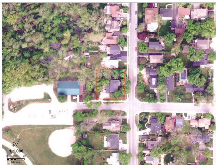
Figure 25: Subject property identified in 2023 aerial photography (Town of Halton Hills 2024)
