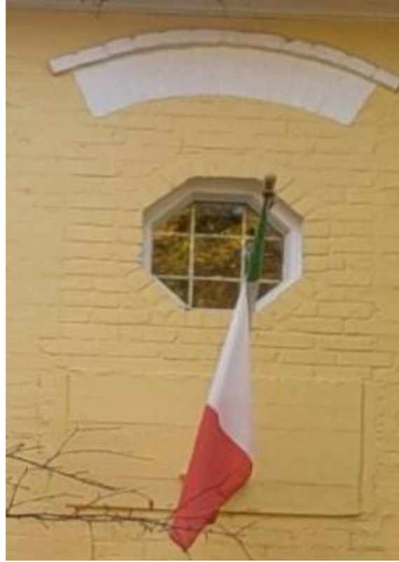
Figure 30: Second storey octagonal window featuring infilled segmental arch and hood mould (Town of Halton Hills 2024)
