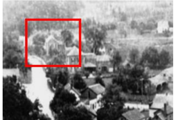
Figure 18: Subject Property identified in c.1910 photograph of Glen Williams' Main Street (EHS p480f)
