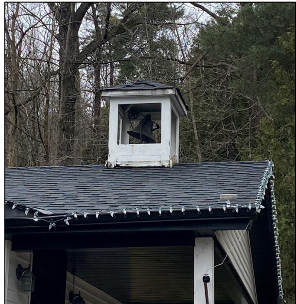
Figure 31: Bell and cupola located on the roof of the contemporary addition (Town of Halton Hills 2024)
