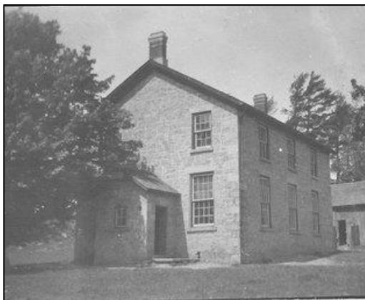
Figure 7: Exterior of Gibraltar Schoolhouse, c.1909 (EHS 21866)
