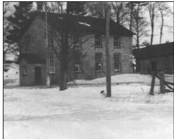
Figure 16: Exterior of Gibraltar Schoolhouse, c.1944 (EHS 11520)
