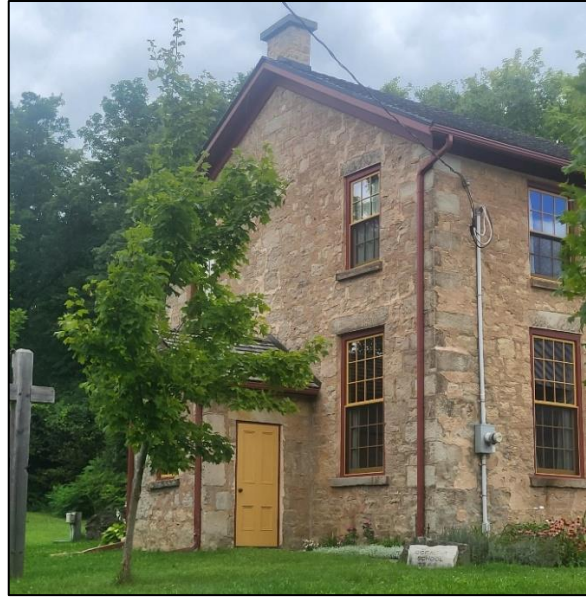
Figure 31: Partial front (southwest) and side (southeast) elevations of the subject dwelling (Town of Halton Hills 2024)
