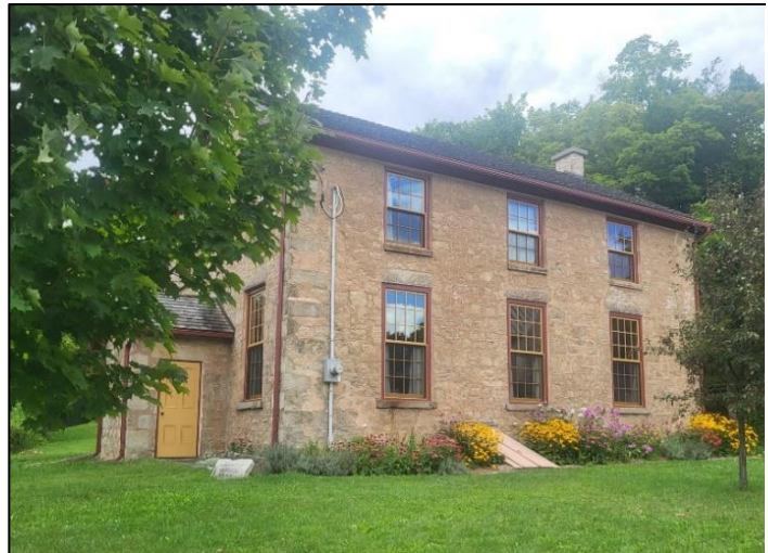
Figure 33: Side (southeast) elevation of the subject dwelling (Town of Halton Hills 2024)
